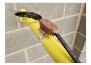
Mount the pre-wired thermostat onto the inlet pipe utilising one of the pipe clamps included with the shower assembly (the inlet pipe is not included).
