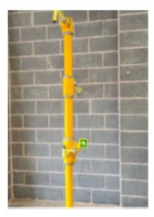
Install the 3 pre-assembled straight lengths of yellow foam insulation using the Velcro fastenings onto the straight large diameter upright pipe lengths, as shown.
