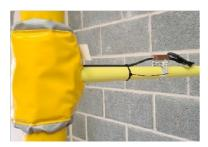
Cover #3 will fit over the main upright tubing of the shower at the horizontal inlet tee, again fasten with the Velcro flaps and drawcords.
