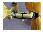
Loop the cable around the valve & back down the opposite side of the pipe to the eyebath valve as shown. Run the cable along the eyewash inlet piping and loop around the valve. Terminate as shown. Depending on where the thermostat is mounted will depend on where the heating cable finishes, ensure the eyewash valve has heating cable around it and complete the heating cable installation by securing the pre sealed end to the pipework. Again, secure the heating cable as previously stated.
