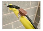
Mount the pre-wired thermostat onto the inlet pipe utilising one of the pipe clamps included with the shower assembly (the inlet pipe is not included).
