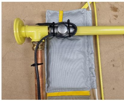
Mount the pre-wired thermostat housing either on to the installation inlet pipework or a suitable close by flat surface
